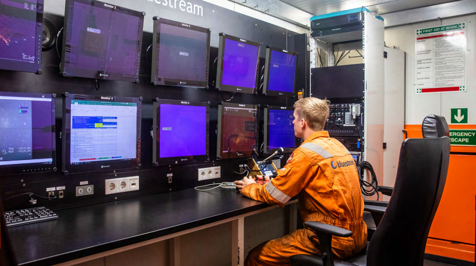
Standard configuration within the ROV control container
